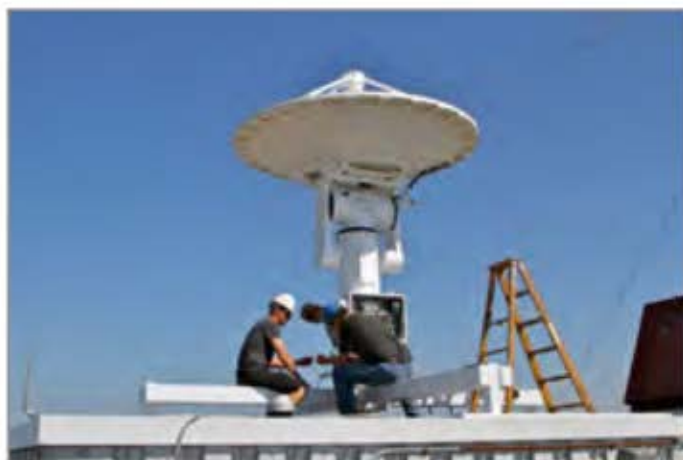
Figure 3. Installation of the SSEC XIL-band Direct Broadcast antenna on the UW-Madison campus in September 2011.
